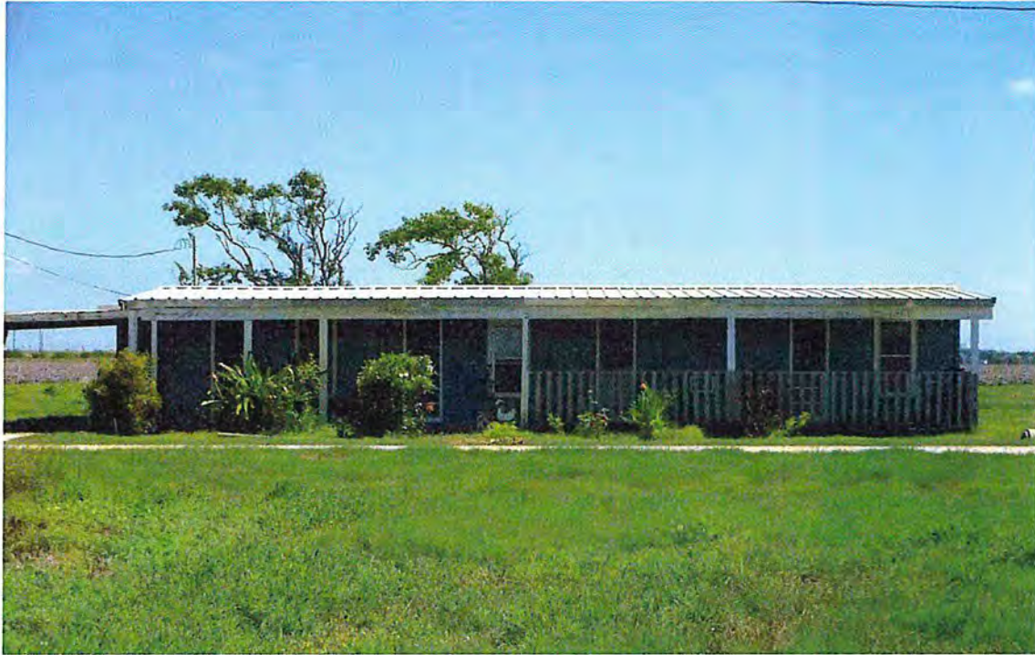
View of Resource 05, facing east
