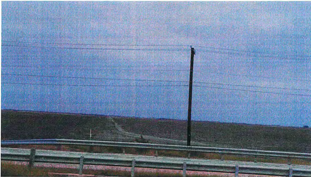
6. Downstream of Outfall 003 proposed location, looking northeast. Highway 181 in foreground. Drainage swale in center.
