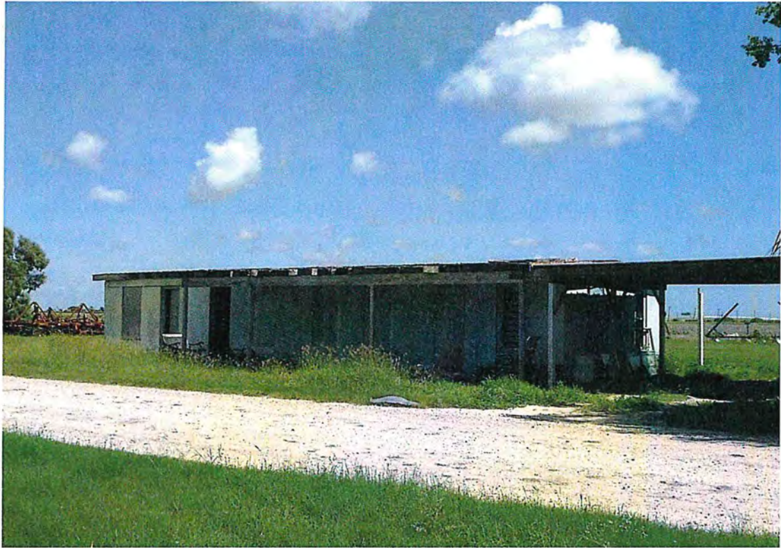
Oblique view of Resource 03, facing northeast
