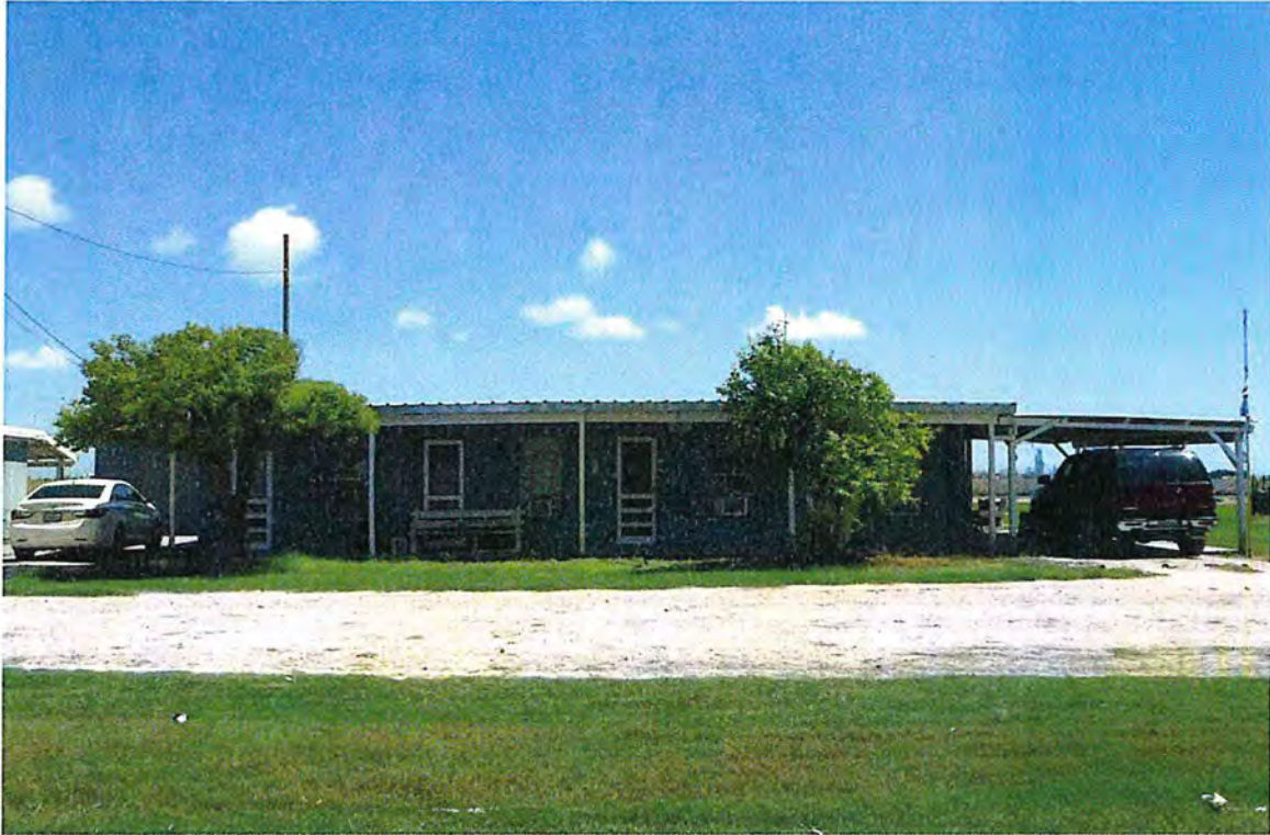
View of Resource 07, facing east
