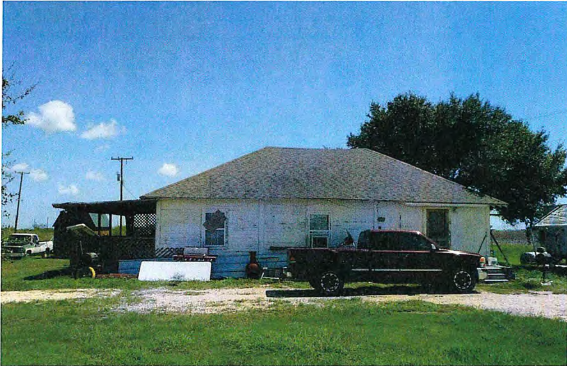
View of west elevation of Resource 01, facing east
