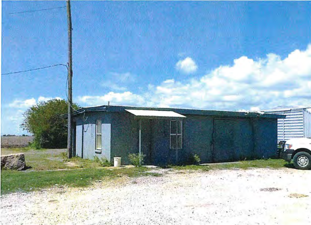
View of Resource 08, facing east
