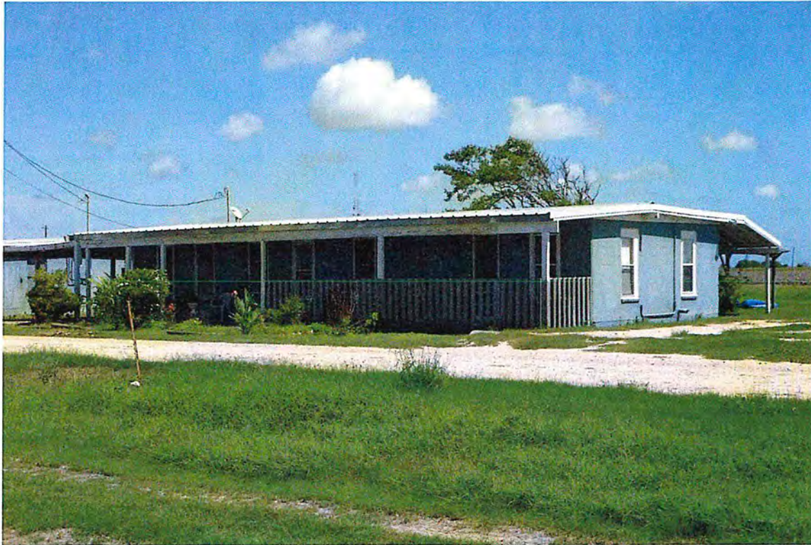
Oblique view of Resource 05, facing northeast
