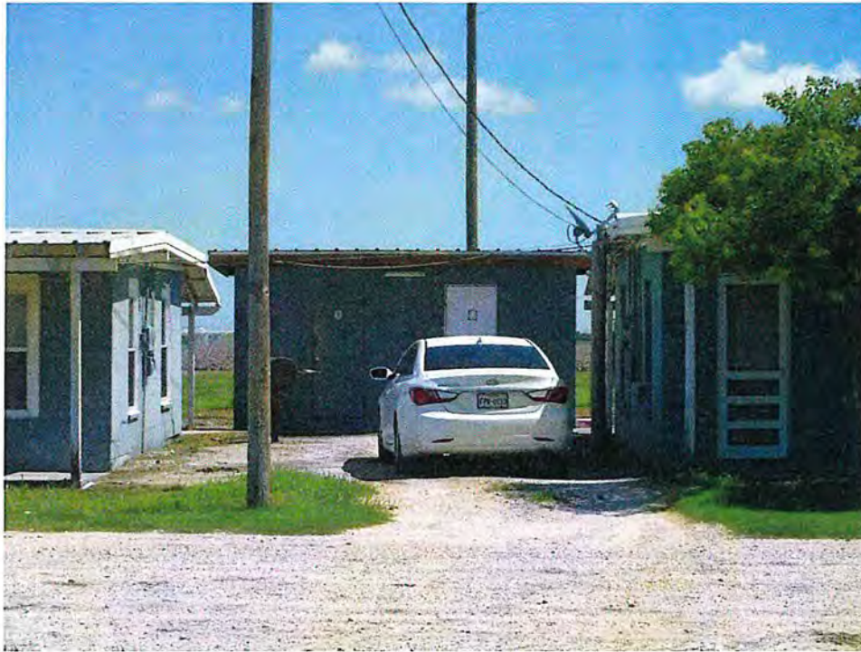
View of Resource 06, facing east
