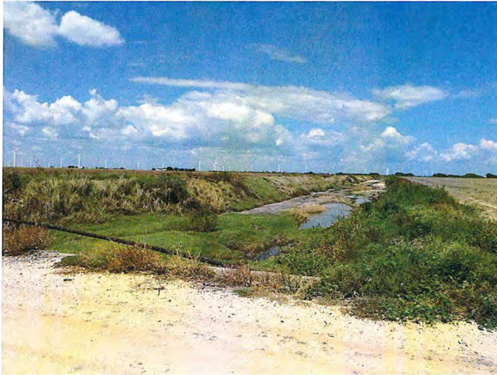
View of canal (Resource 02), facing north
