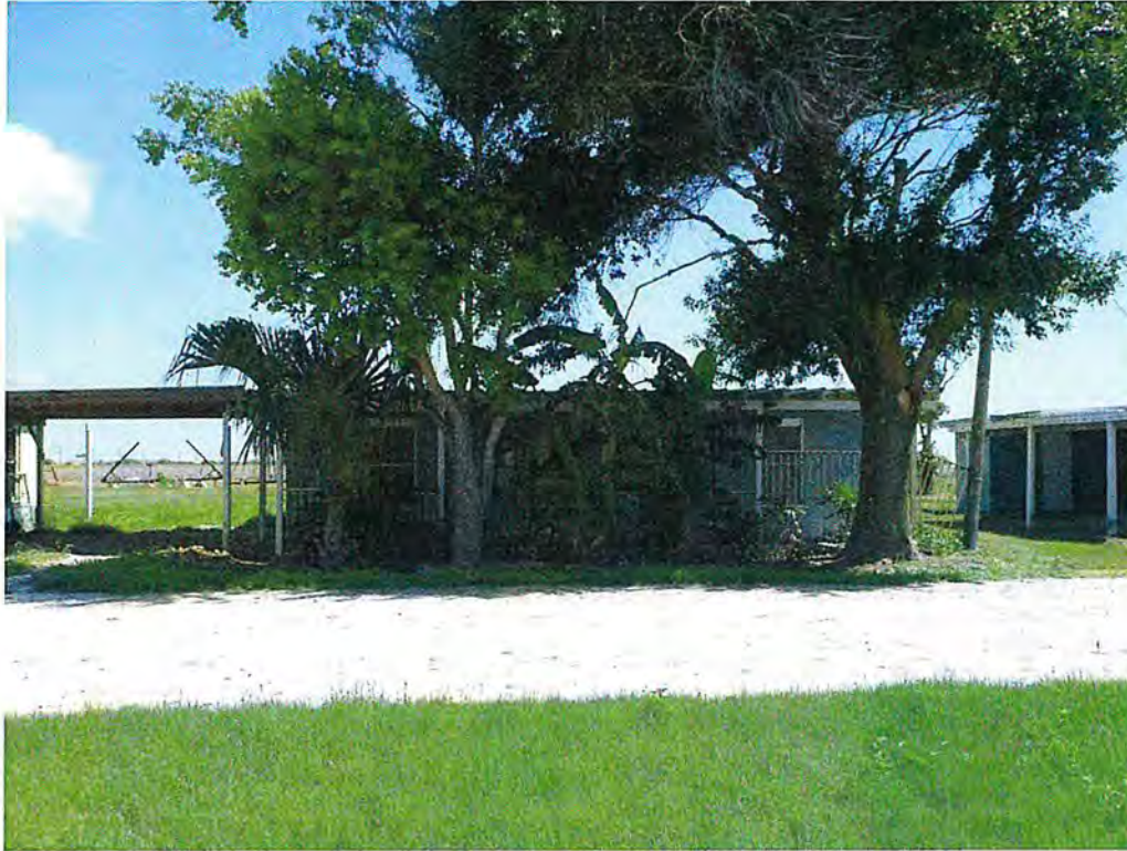
View of Resource 04, facing east
