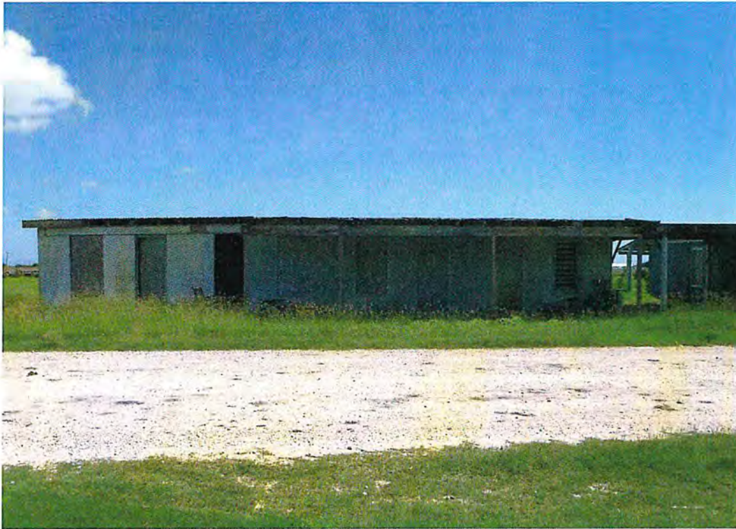
View of Resource 03, facing east
