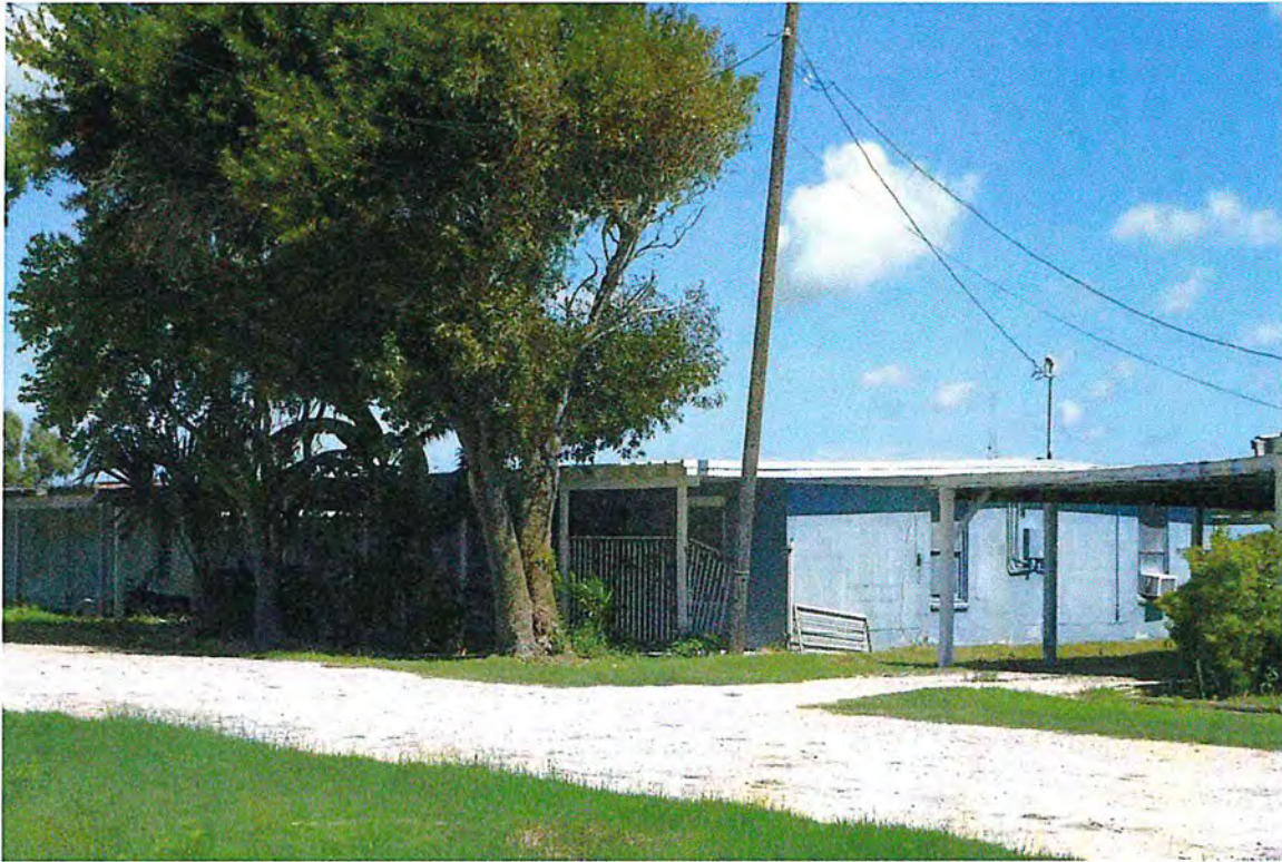
Oblique view of Resource 04, facing northeast
